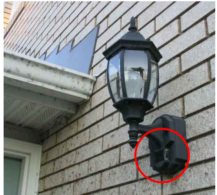
Photo and motion sensors are integral to the light, as shown in the red circle above.
